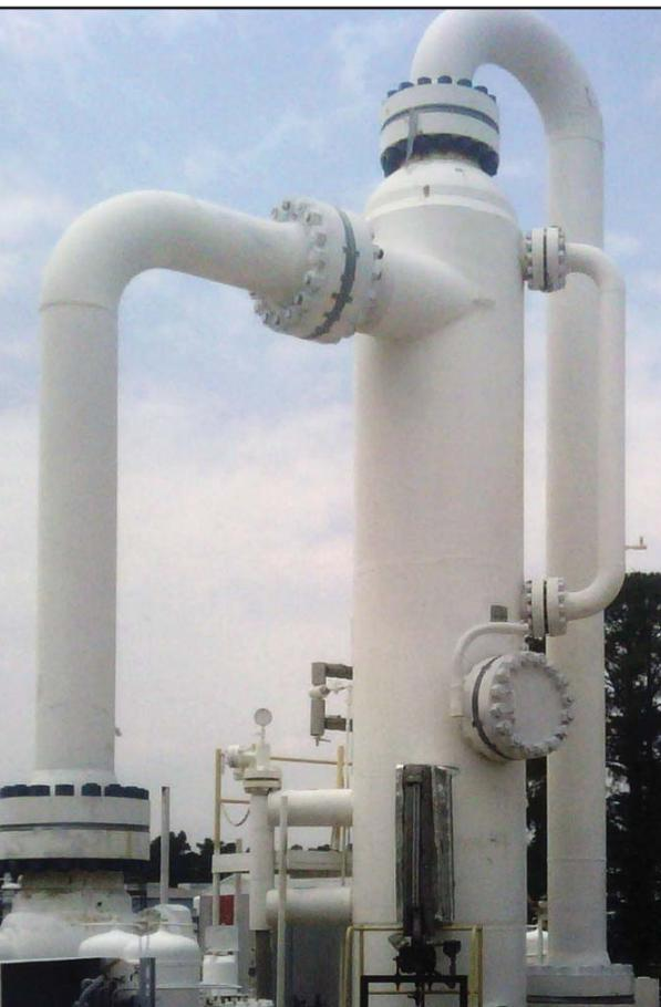
The “Vortex Cluster” is suited for gas dominant, liquid dominant, or liquid/liquid separation. Lower retention times and dramatically improved separation are the result of fluid control. This results in a smaller new vessel, improved separation, and increased flow through existing vessel with a Retrofit. No foam, up to 90% turndown.
